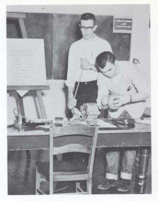
If your electric motor is dirty, see these boys! Larry Sloup is demonstrating the proper way to clean an electric motor as Don Romshek explains each different step.
