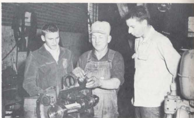
Henry Sobolik, of Mayfield Implement Company , is showing Jerry Meister and Fred Bock the way to overhaul a tractor motor. Mr. Robert Mayfield is owner of this company.
