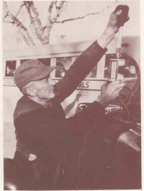
Robert Doner uses the anti-freeze gauge to see if the school bus meets specifications for winter weather.
